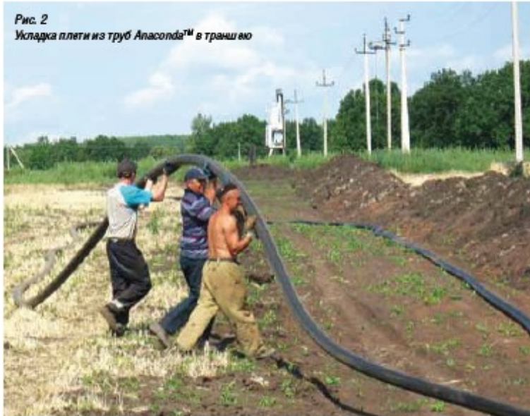
Fig. 2 Laying a stalk of Anaconda™ pipes into a trench
