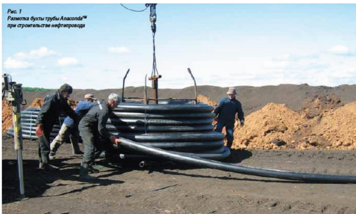
Figure 1 Unreeing of Anaconda™ pipe reel during pipeline construction
